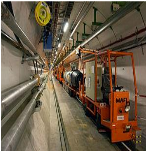
Figure 3: The former LEP tunnel at CERN being filled with magnets for the LHC.
