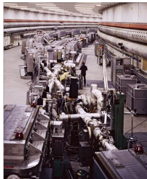
Figure 2: This view of Intersection 5 (15), (fig.1), in 1974 clearly shows the layout of the magnets and the crossing of the two beams pipes.
